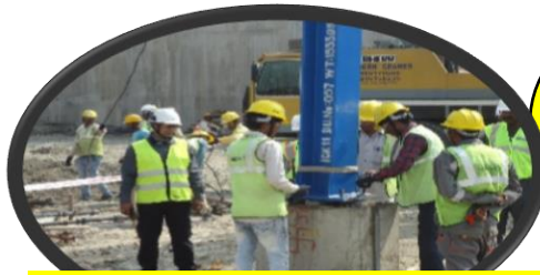
First Column Erection
