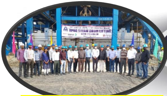
Steam Drum Erection
